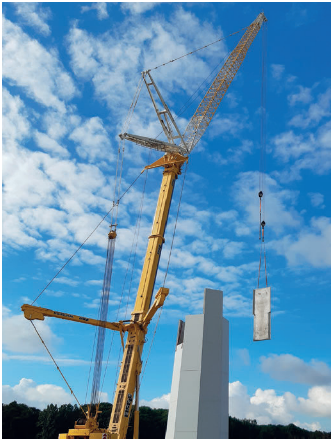
Fig. 8: Ventur 4.0 assembly work
