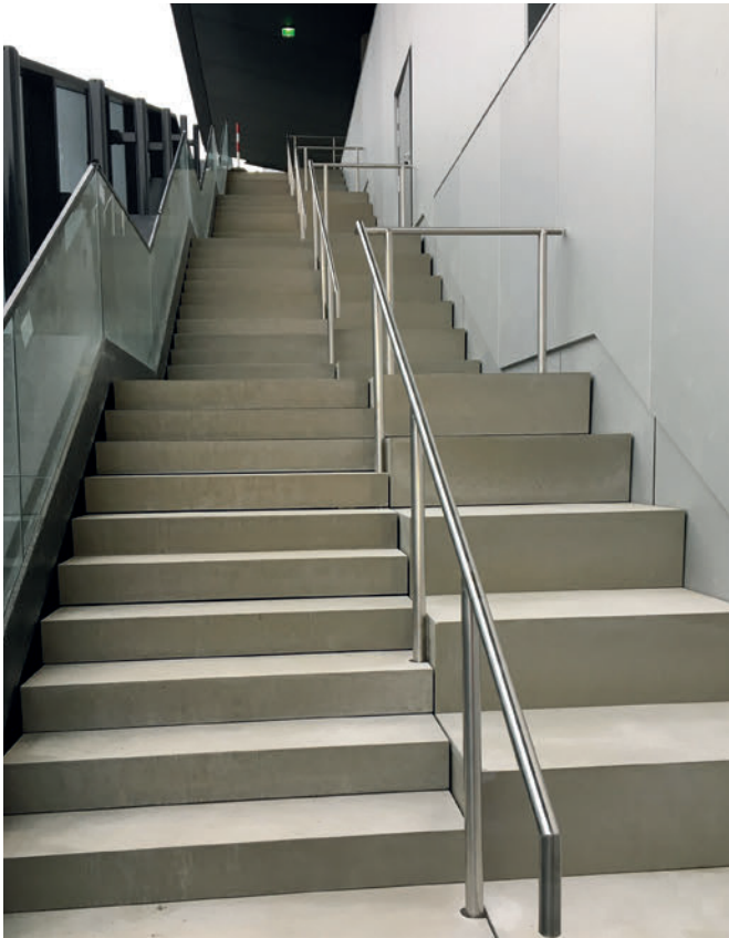
Fig. 3: New Axel Springer Building, Berlin
