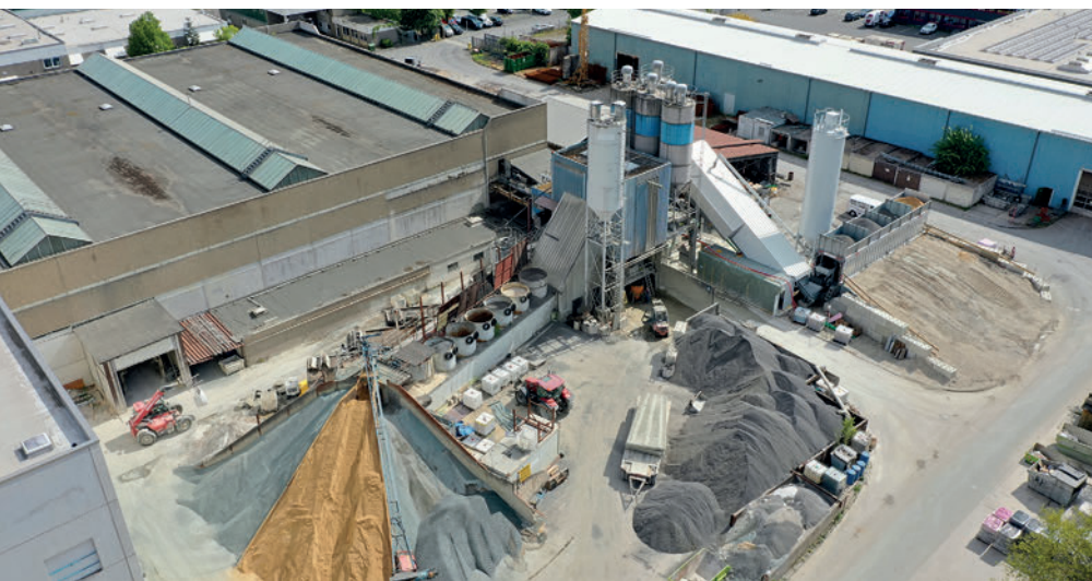
Fig. 7: Ventur concrete mixing unit, Siegen
